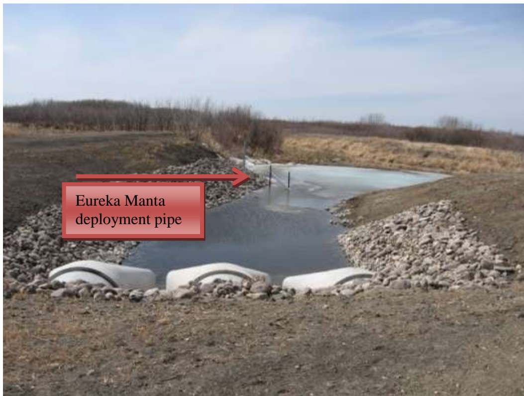
A5 outlet (new Thief River/SD83 outlet structure).
